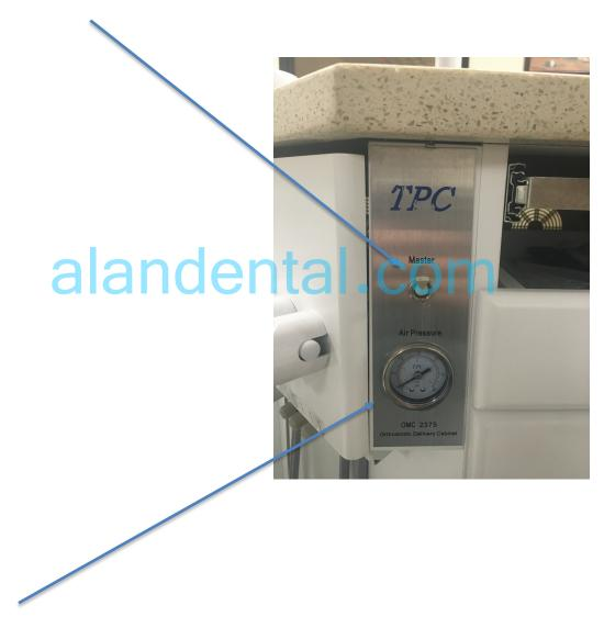
B. HANDPIECE PRESSURE GAUGE: Indicates pressure adjusted by the Drive-Air Control Knob. Avoid exceeding the manufacturer's recommended handpiece pressure. (30 - 35 PSI for most Highspeed Handpieces)
